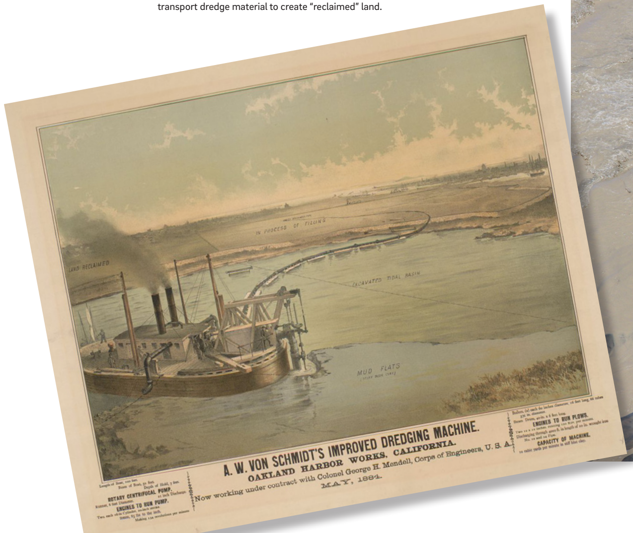
(Bottom left) A.W. Von Schmidt's dredge in 1884, shown dredging blue clay from mud flats in Oakland Harbor. The pipe extending from the dredger to landfill in distance was used to transport dredge material to create "reclaimed" land.
